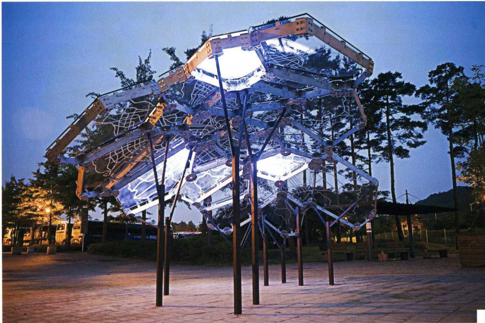
1,2. Every 15 minutes, the Living Light pavilion's LED lighting system goes dark and regenerates patterns based on Seoul's air quality.
