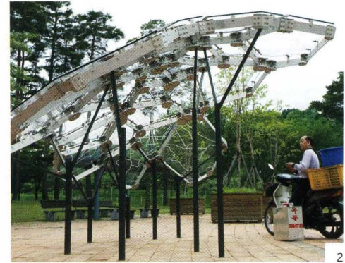
1,2. Every 15 minutes, the Living Light pavilion's LED lighting system goes dark and regenerates patterns based on Seoul's air quality.
